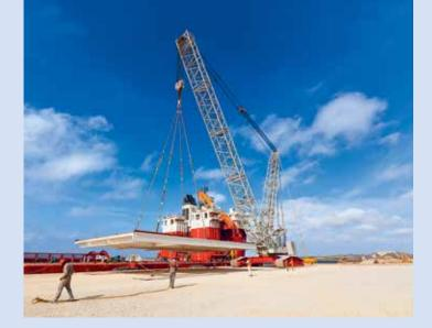
Work to extend the jetty and assemble Africa's largest crane (2,500 tons of lifting capacity) at the Paenal yard.
